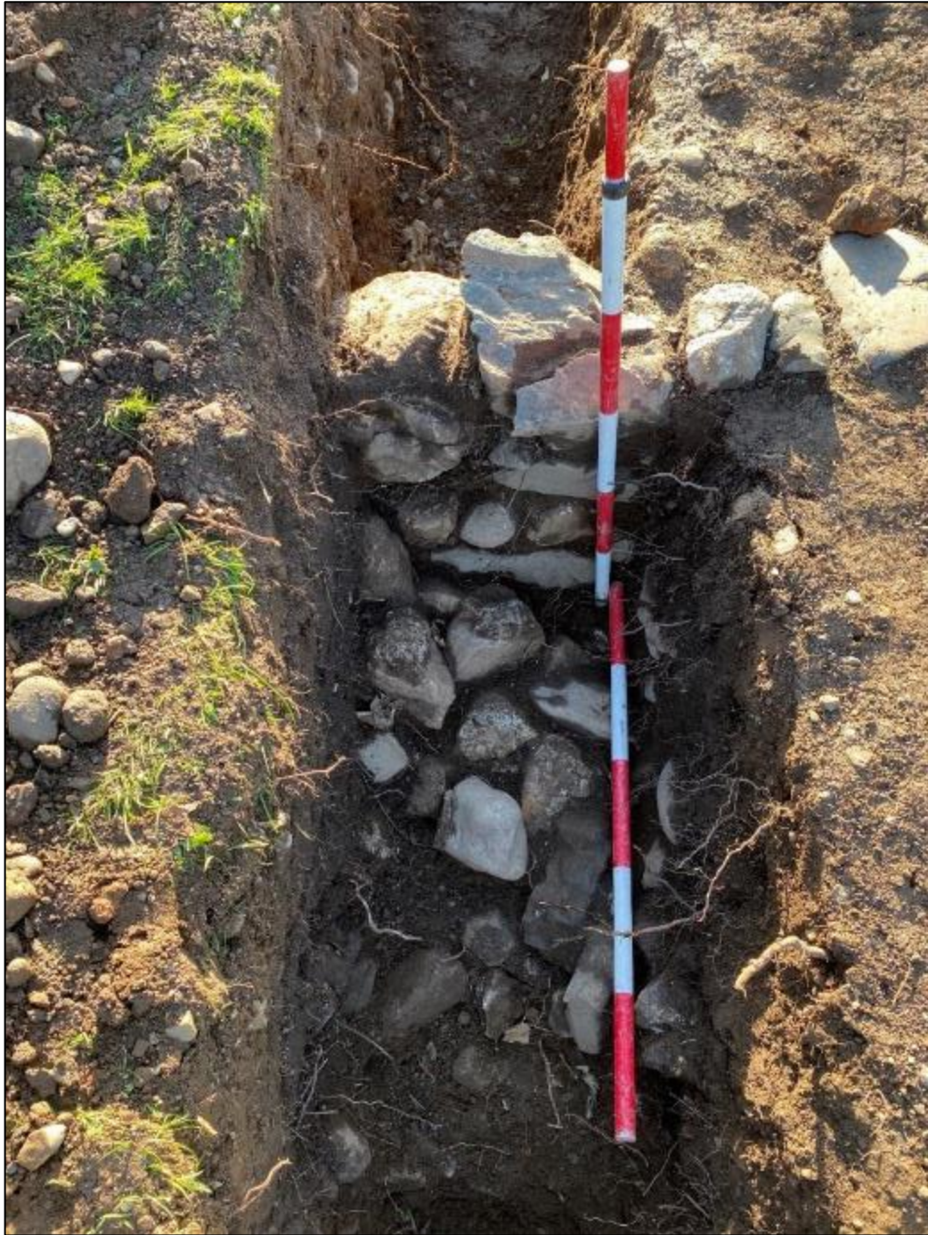
Plate 19: View of the front face wall C.04 uncovered in Cutting 1
